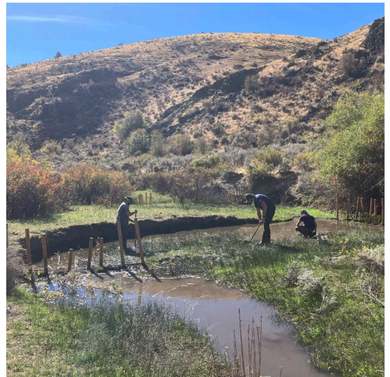
Beaver dam analog construction by WCC Crew. Photo by Kurt Merg, WDFW.
