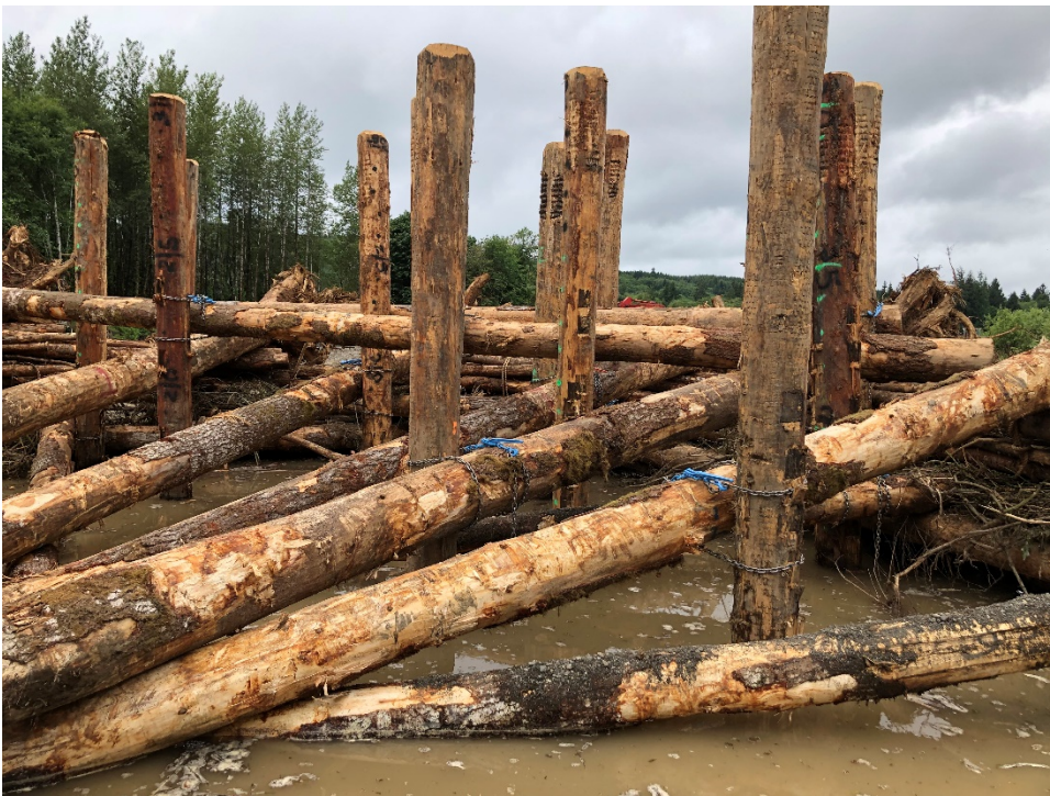
Engineered log jams help stabilize stream banks and keep our rivers healthy, improving the survival of salmon and other native fish and wildlife.
