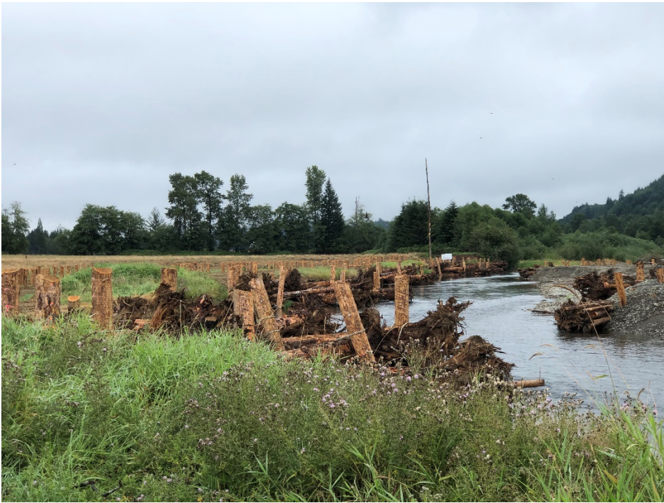
Engineered log jams help stabilize stream banks and keep our rivers healthy, improving the survival of salmon and other native fish and wildlife.
